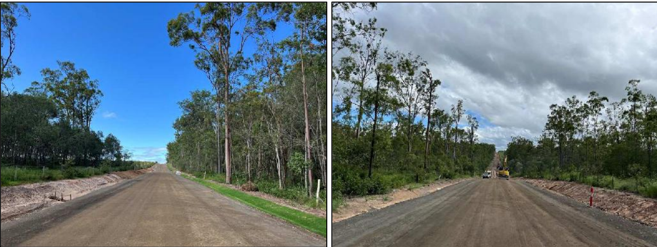
Photo set 2: Remediated vegetation damage along Bushland Road
